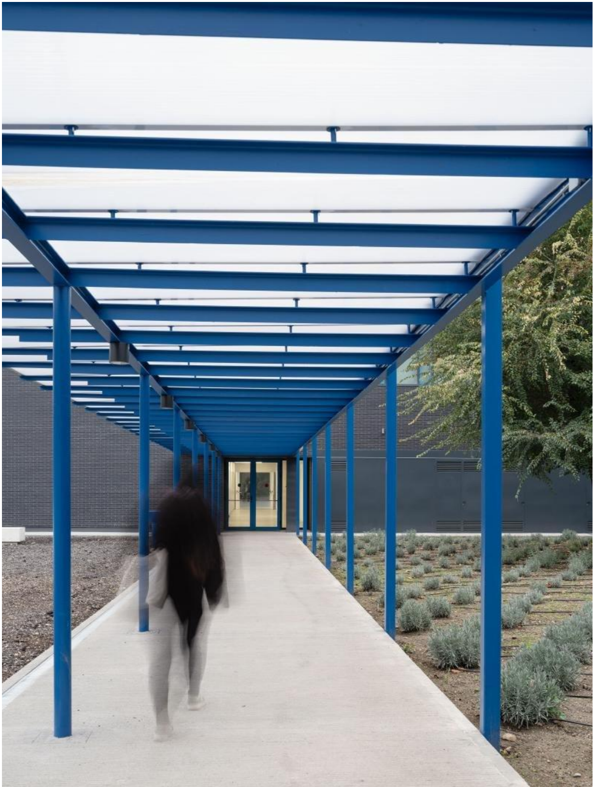
Figure 16 - Galerie ouverte, School of Arts Valladolid, Espagne © Luis Diaz Diaz
